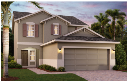
ELEVATION 3 - STUCCO FINISH
